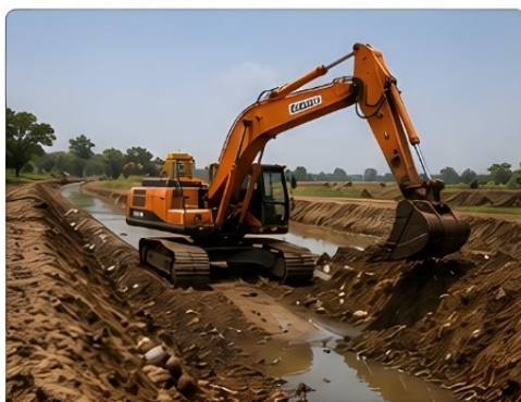
CANAL DESILTING WORK
